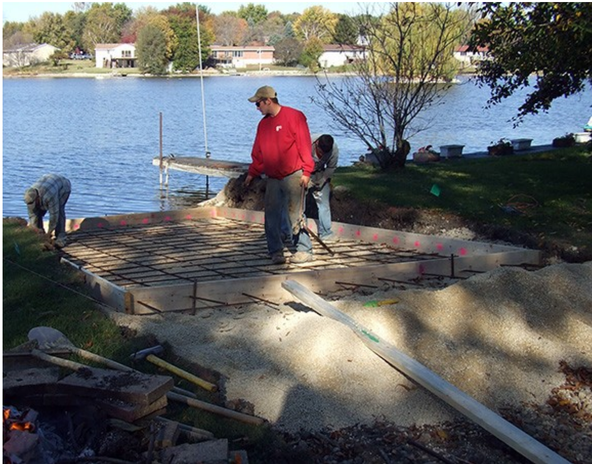
Rebar was installed.
