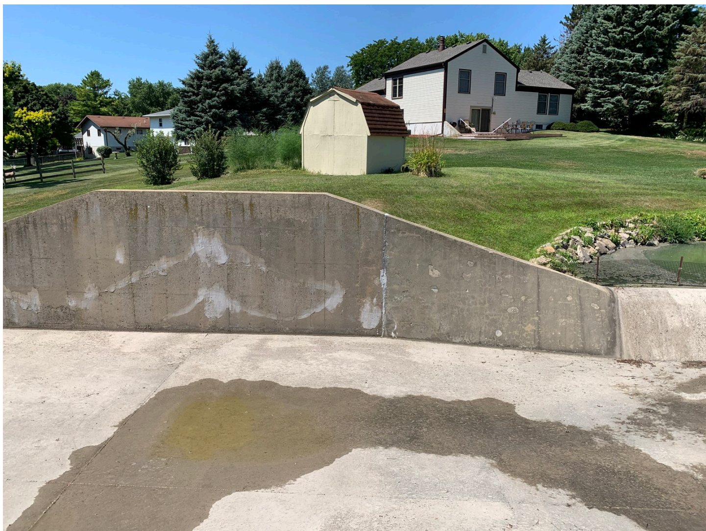
Photo #1 – West emergency spillway wall. Good condition.
