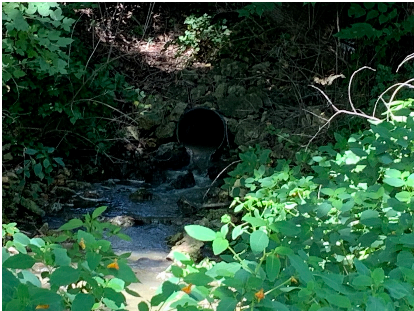
Photo #9 – Principal spillway outlet pipe.
