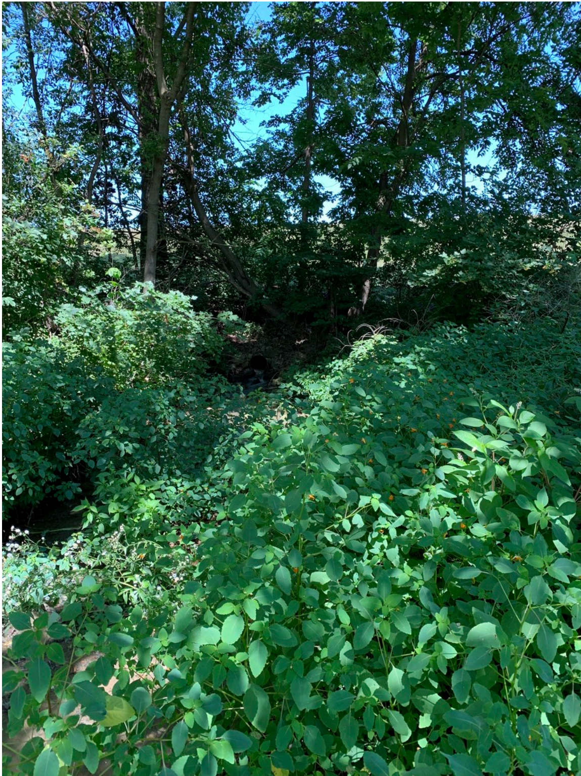
Photo #8 – Principal spillway outlet and channel.
