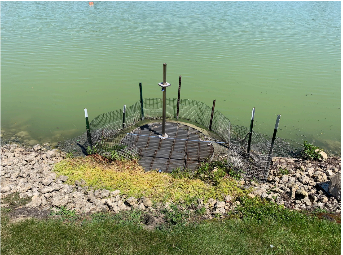
Photo #7 – Principal spillway. Good condition.
