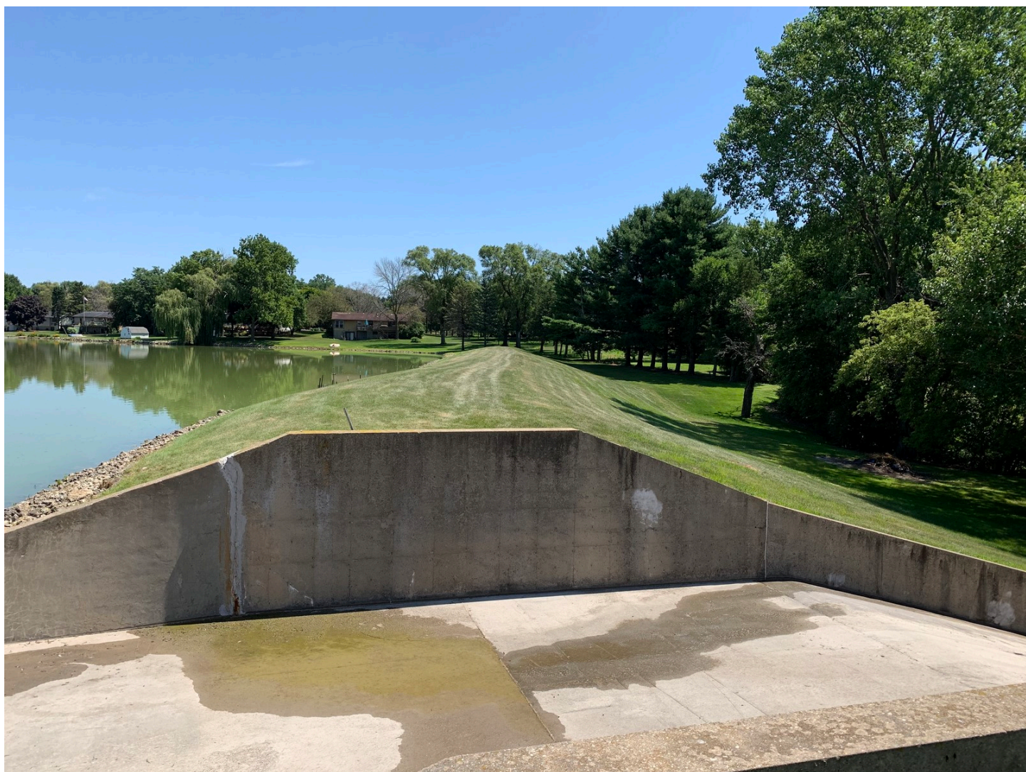
Photo #10 – Dam looking east. Good condition.
