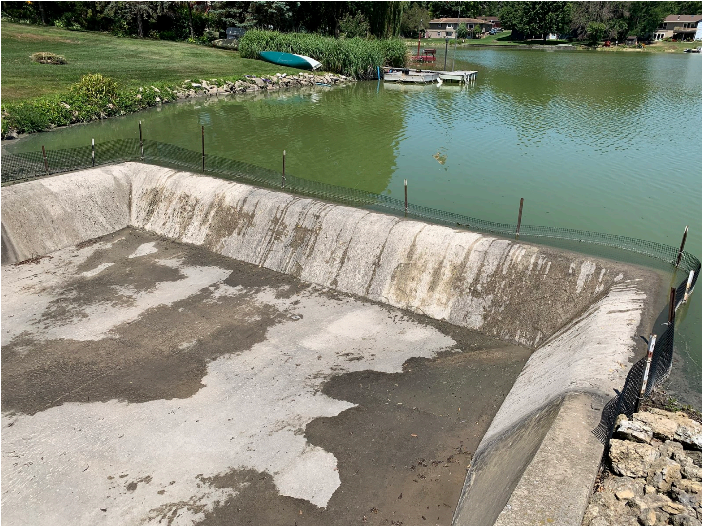
Photo #3 – Inlet side of emergency spillway. Good condition.
