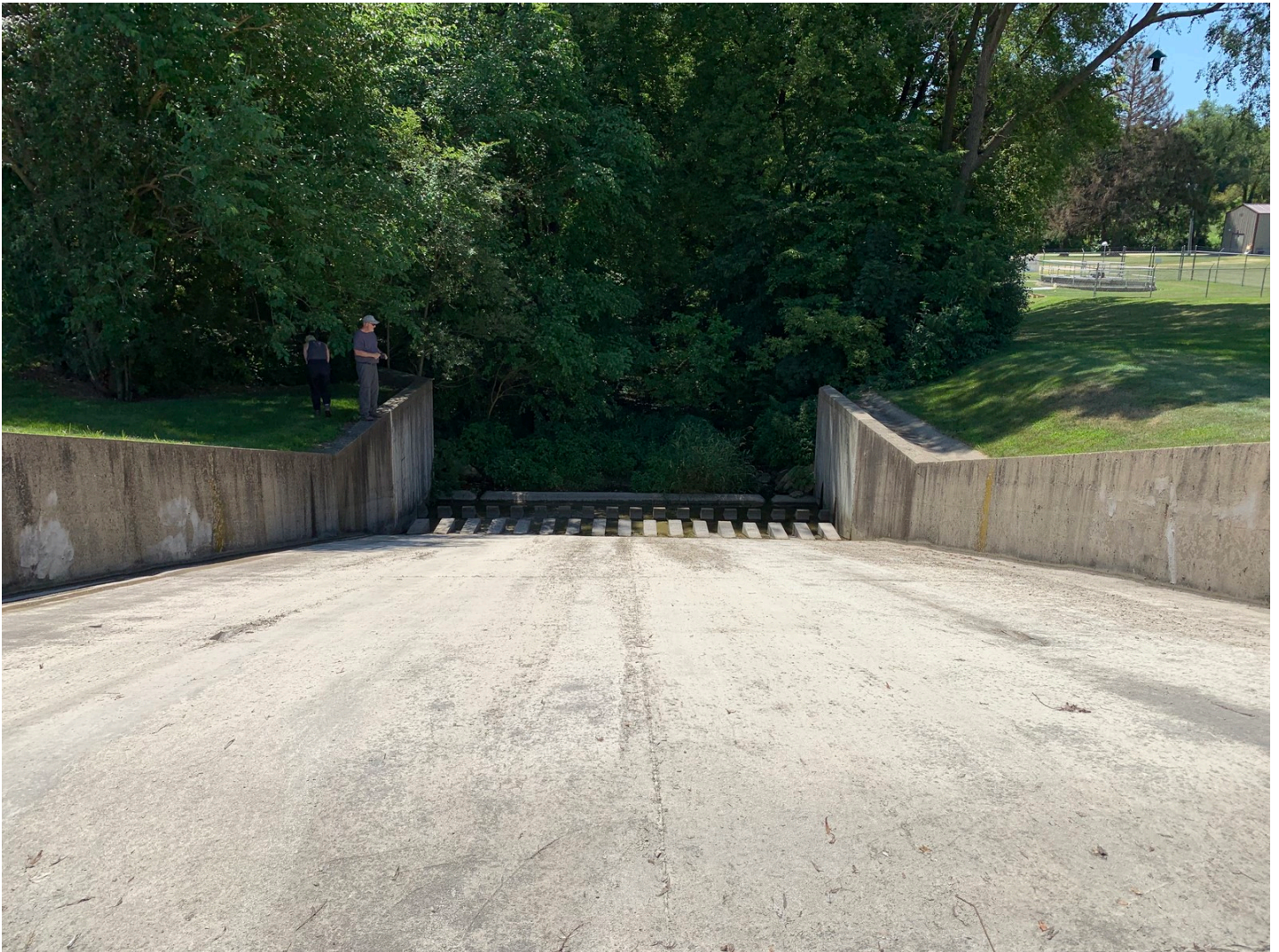
Photo #4 – Downstream end of emergency spillway. Good Condition.
