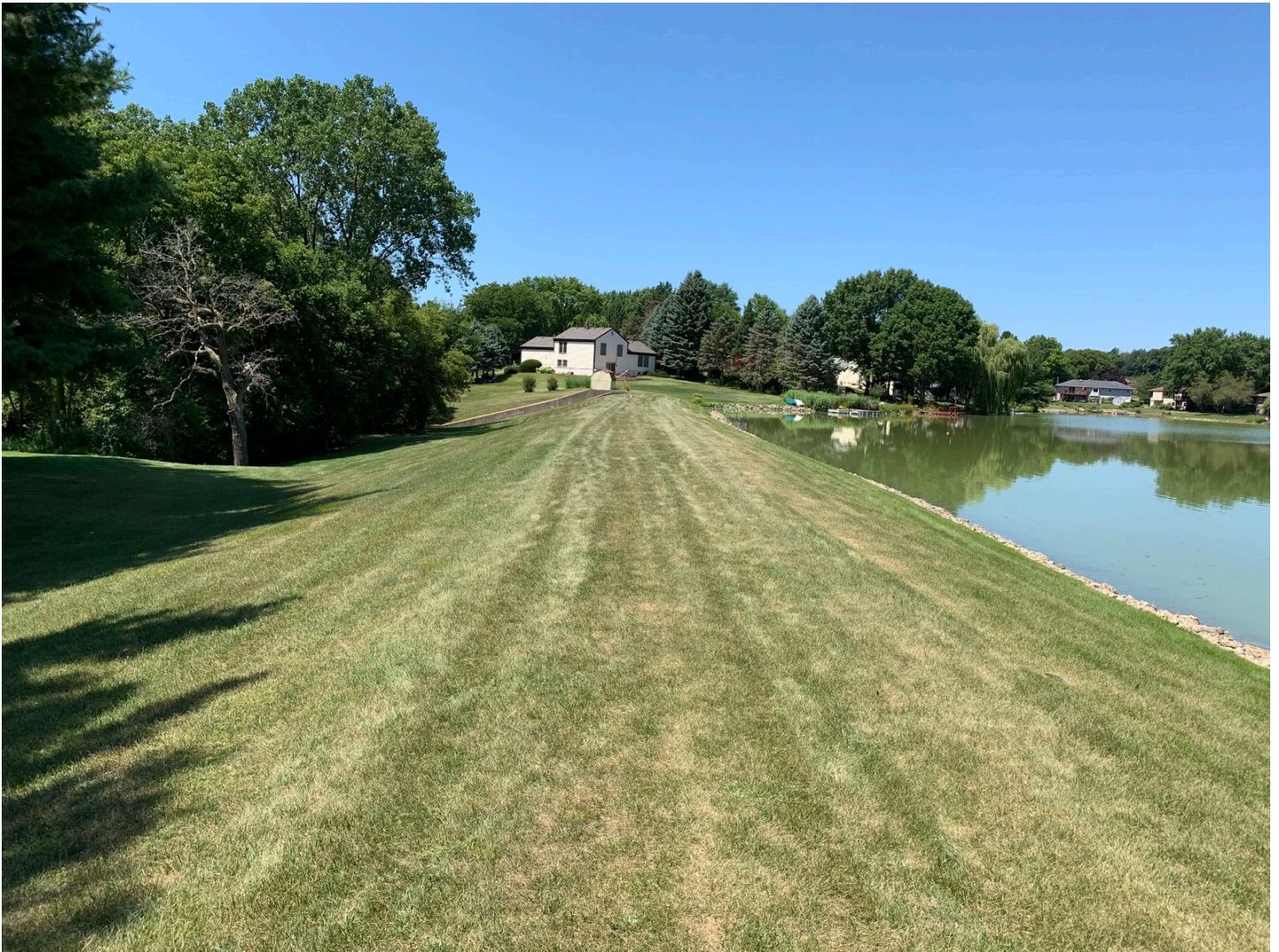
Photo #11 – Dam looking west. Good condition.
