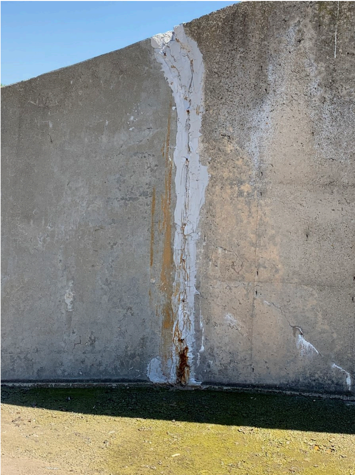
Photo #2 – East emergency spillway wall. Repaired joint, good condition.
